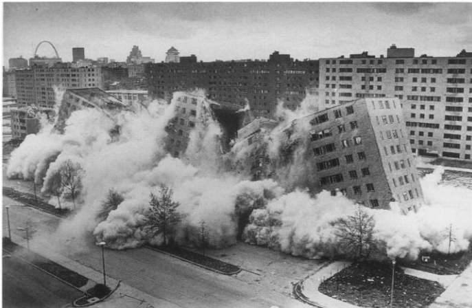
1. Pruitt-Igoe demolition. (Courtesy St. Louis Post-Dispatch)
